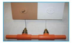
Capilary tubes run above the ceiling and enter the fire zone through a small hole in the cornice
